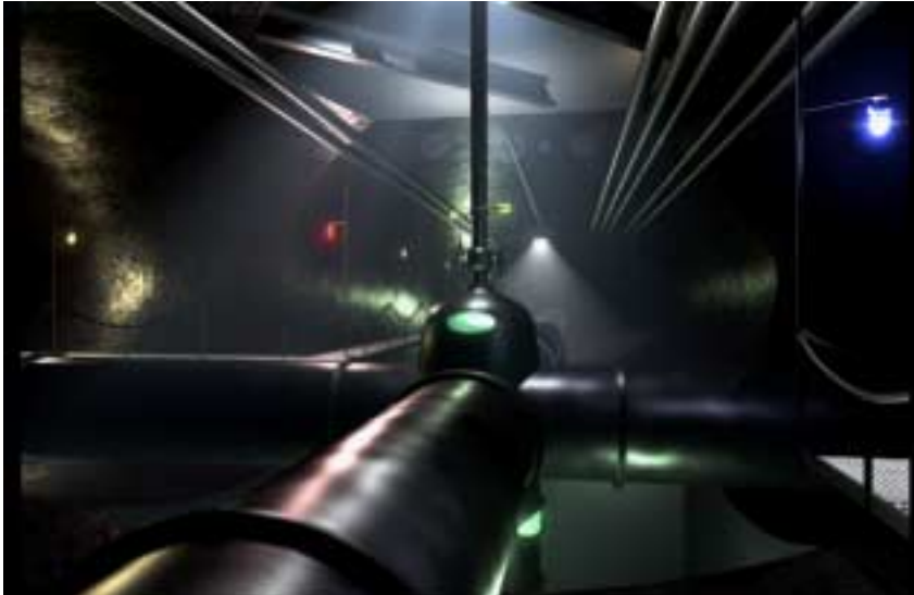
Wide view of pipes and tunnel
